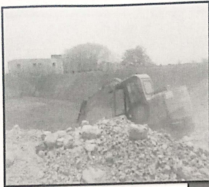
Earthen Water Pond
